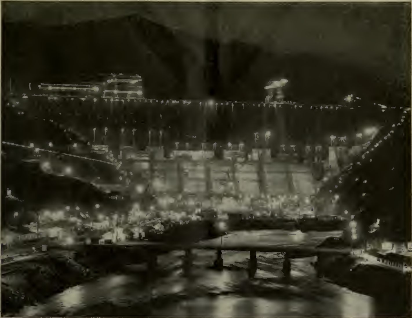
Night construction at TVA's Fontana Dam on the Little Tennessee River in western North Carolina
